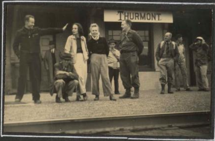
TIME TO SPARE AT THURMONT
