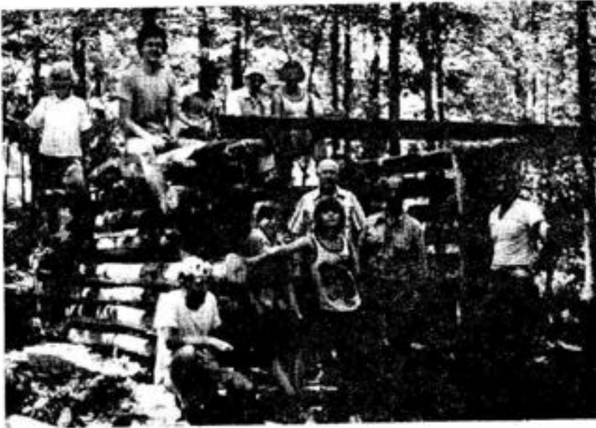
MCM Workers Showing Progress Made on Shelter During June Work Trip
